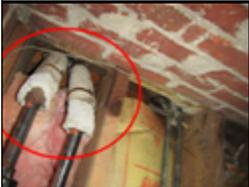
Some insulation material on the boiler distribution pipes is of an age and material type that could be considered as a presumed asbestos containing material (PACM). It is recommended that an Environmental Testing company licensed for Asbestos be consulted to evaluate the significance of this concern and make recommendations for testing, removal or repairs.
